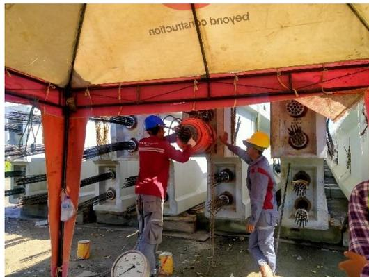
**Gambar 4. 16** Proses Stressing Balok Girder
