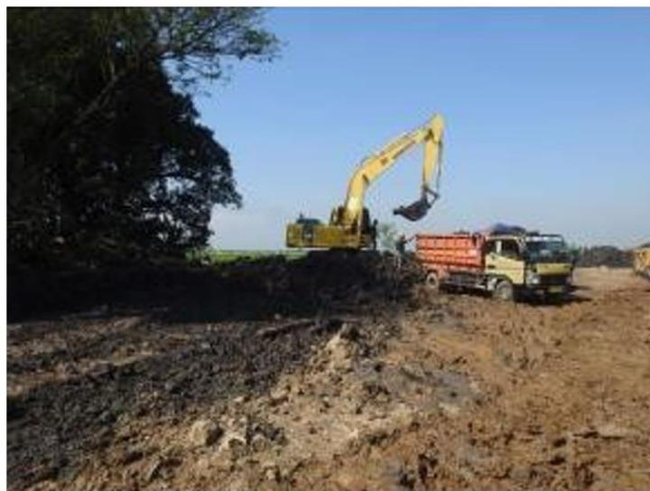
**Gambar 4. 5** Loading tanah ke *Dump Truck*
