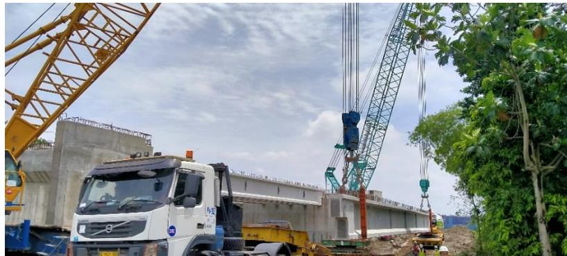
**Gambar 4. 19** Proses *Erection Girder*
